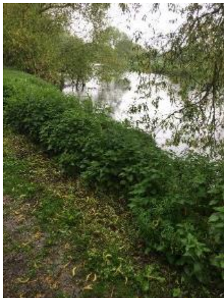
Photo of Edge Protection
